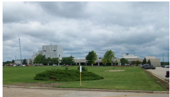
Continental Dairy Facility in Coopersville, MI
