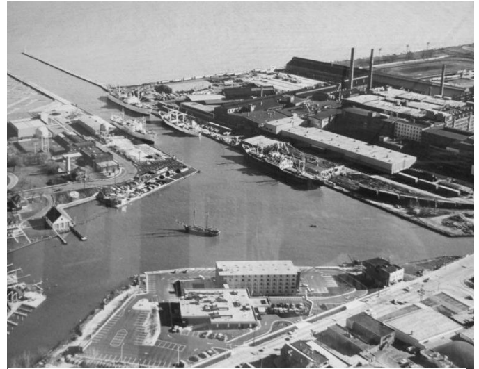
Kenosha Lakefront Plant before it was demolished.
